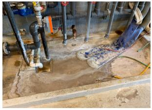
Exposed concrete areas are heavily stained in areas and could potentially be damaged from the various drains
