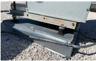
Ductwork located on the roof was not properly supported after the last re-roof or roof repair.
