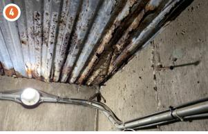
Water seeping into tunnel causes rust and panel separation from ceiling
