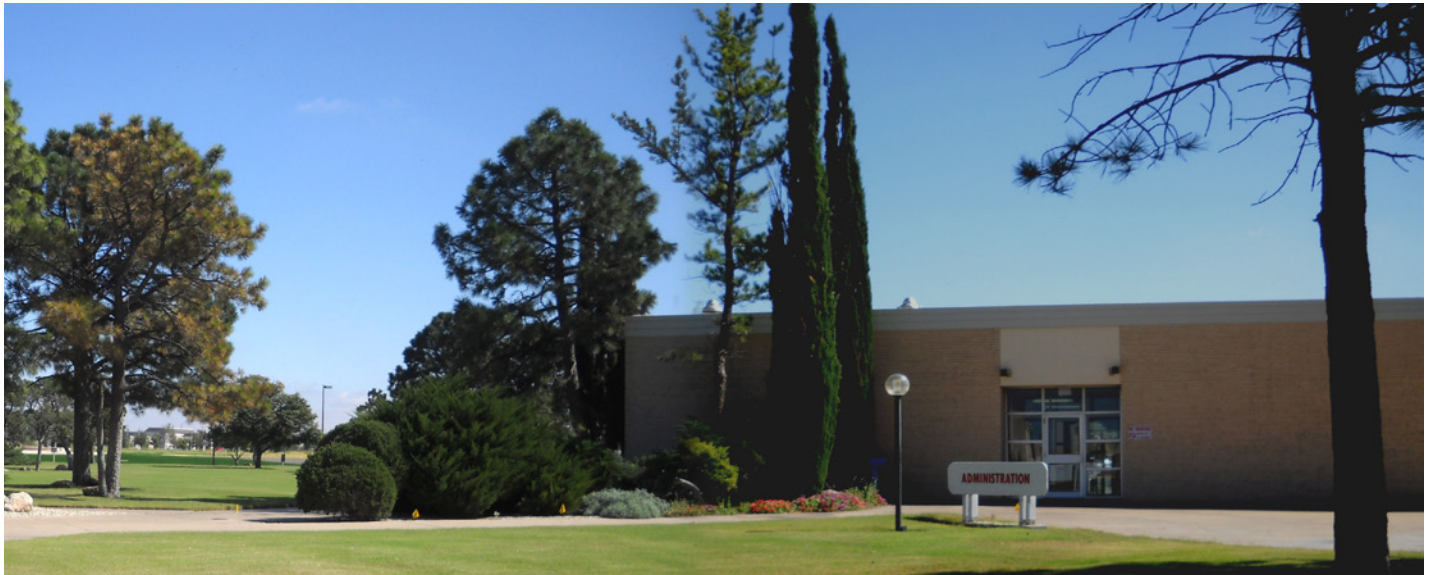
Administration Building, NMJC Campus.
