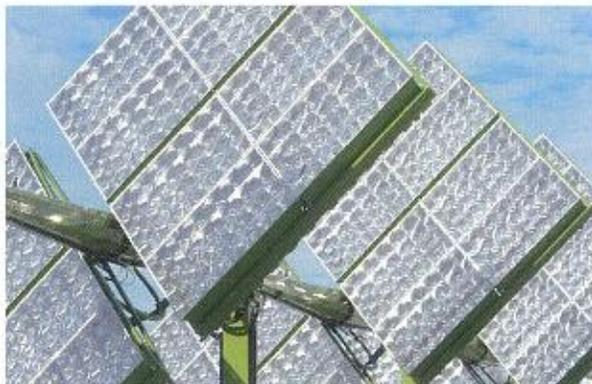
The Green Volts CPV System is currently being used for utility scale installations in excess of 2mW. One benefit to using CPV is that the cells do not lose efficiency due to high temperatures. Traditional PV panels see a decreased drop in efficiency when temperatures rise. The Green Volts CPV remains efficient regardless of outside ambient temperature. The Green Volts CPV
